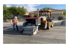
Staff continues to make new installs a priority as they are received. 19 new water services were installed this month. The photo below shows staff using the asphalt zipper to grind the asphalt allowing for trench excavation.
