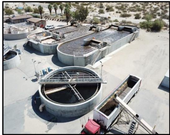
Staff installed two new baffles on the center well of Clarifier 3. The placement of the inlet for Clarifier 3 has always been a bad design that would cause mixed liquor to get pushed at a high velocity out of the clarifier and straight to the ponds via the weirs. By adding these two stainless-steel baffles, staff has slowed down the mixed liquor velocity and solved this issue.
