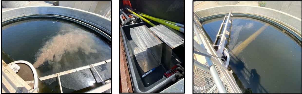
Staff encountered an issue with RAS Pumps 3 and 4. These pumps had a 10-foot rag pulled into it and most of the piping had to be dismantled to remove the rag.
