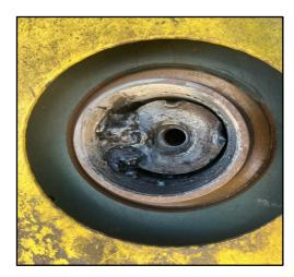
Staff completed a confined space entry into the grit vortex to remove a blockage in the sump pump. Staff removed the paddles, grit, and rags causing blockage, allowing the vortex to return to normal operation.
