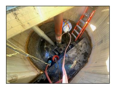
Staff worked on replacing the horizontal auger for the belt press. This project was part of a Capital Improvement Project to replace the components of the auger such as the gearbox, augers, bearings, shafts, etc.
