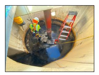
Staff had All Valley Crane come out to pull out the auger at the headworks to replace the brush on the auger. While the crane was here, staff replaced the spider couplings in aerators 8 through 11 on aeration tanks 4 and 5.
