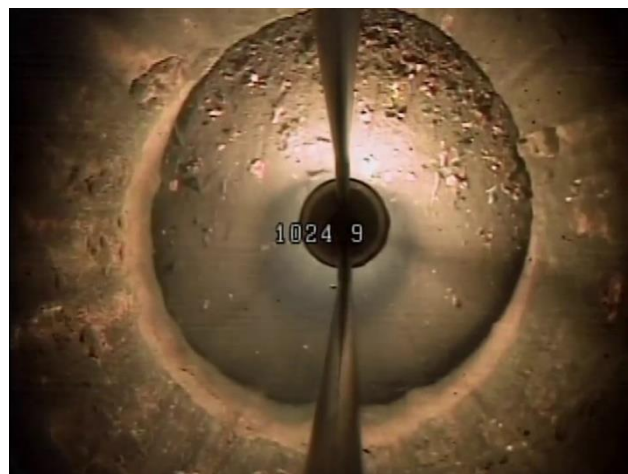
Figure 6 – Accumulated fill in well sump.
