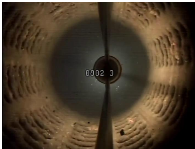
Figure 5 – Encrusting and biological material on louvered openings.
