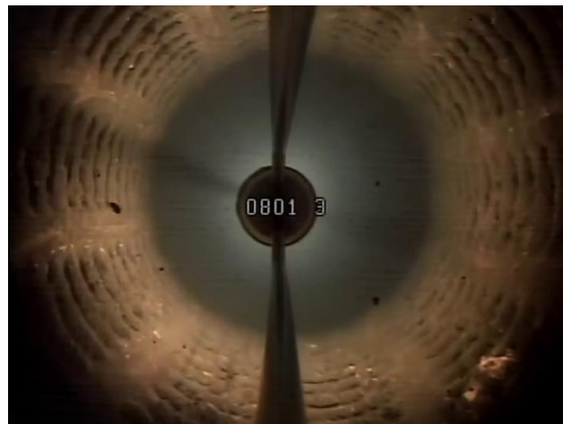
Figure 4 – Encrusting and biological material on louvered openings.
