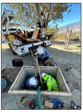
Well 22 Electrical – Staff experienced a few electrical circuit trips at Well 22 in August 2024. Upon further investigation, the wire were not properly torqued, thus creating an excessive heat issue on one of the electrical phases (B-Phase). All wires were re-torqued to proper specifications and the load/heat is now evenly distributed. The random electrical circuit trips have ceased, and the well/motor is operating properly.
