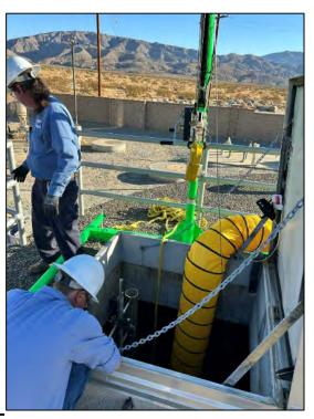
Well 25 Header Leak – Construction & Maintenance staff made a repair to the header due to some misalignment issues and a recent leak. Below are some photos of the header prior to the repair.
