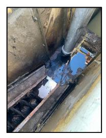
At the main gate of the WWTP, a water line that feeds the laboratory and north building had sprung a leak under the asphalt. Staff hydro excavated a new trench due to the depth of the broken pipe and replumbed a new service line at a more manageable height.
