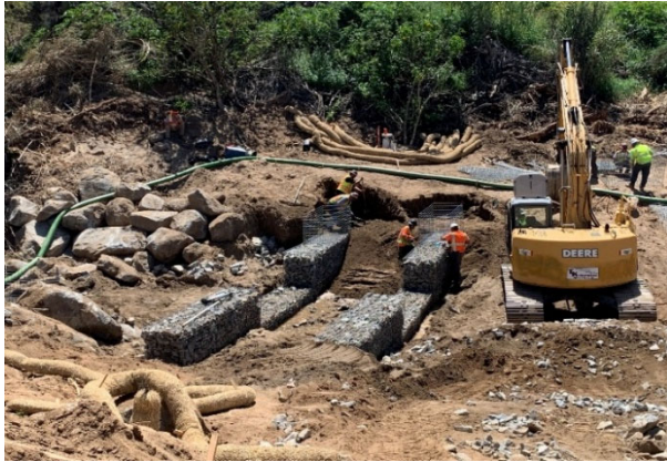
Left: Repair work to protect Western Municipal Water 60 inch steel watermain from erosion damage in 2020. Work was performed on an emergency basis Right: 12-inch CMLC steel cross installation for the City of Norco potable water system. Work was performed in 2021 and was part of a formal bid process.
