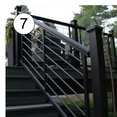
Aluminum Railing and Composite Decks
