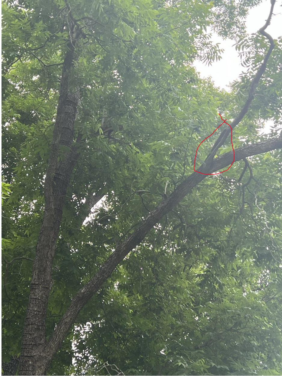
A previous branch that had fallen now has a rot cavity leading into the large branch
