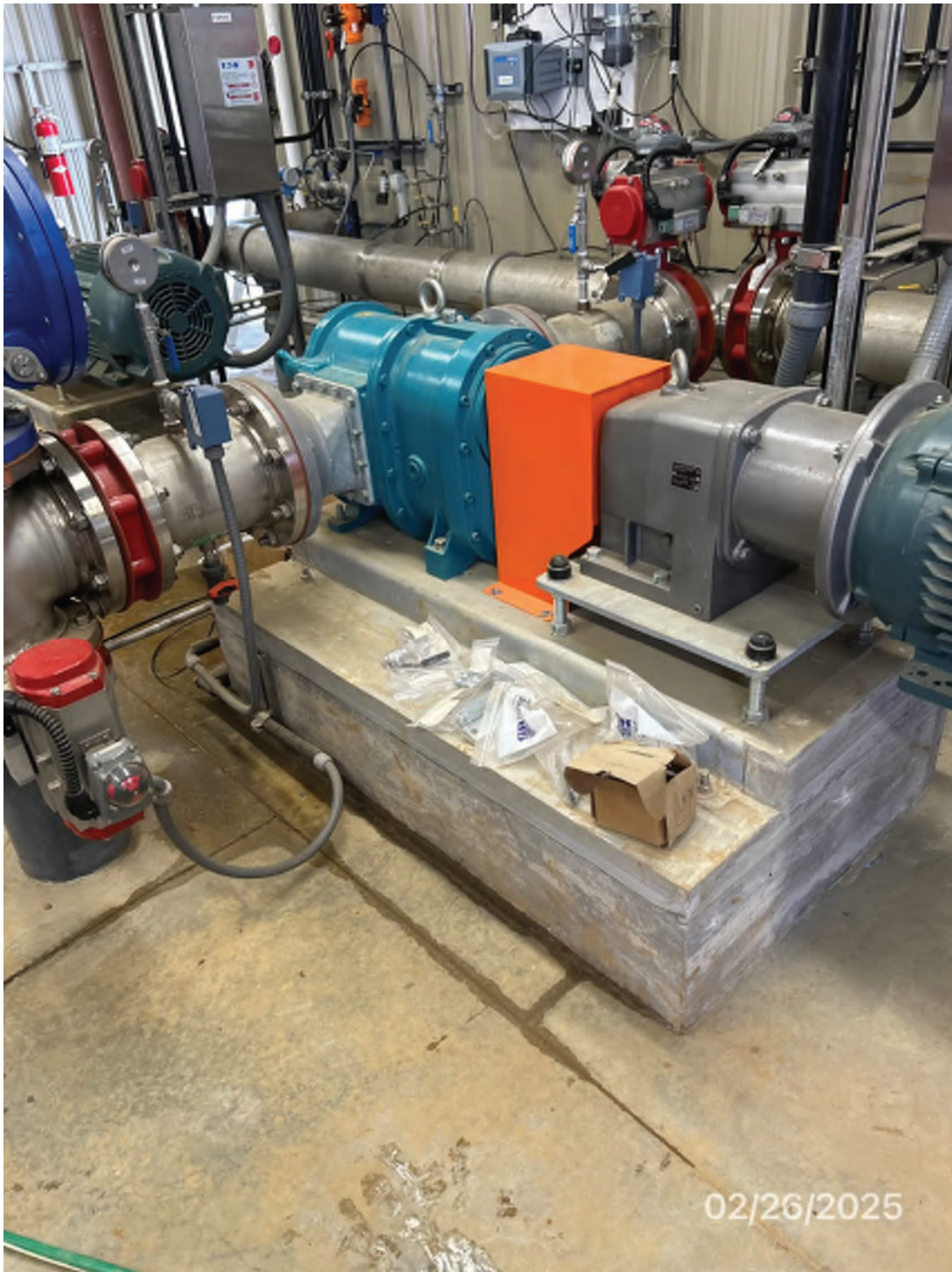
6. Membrane permeate pump
