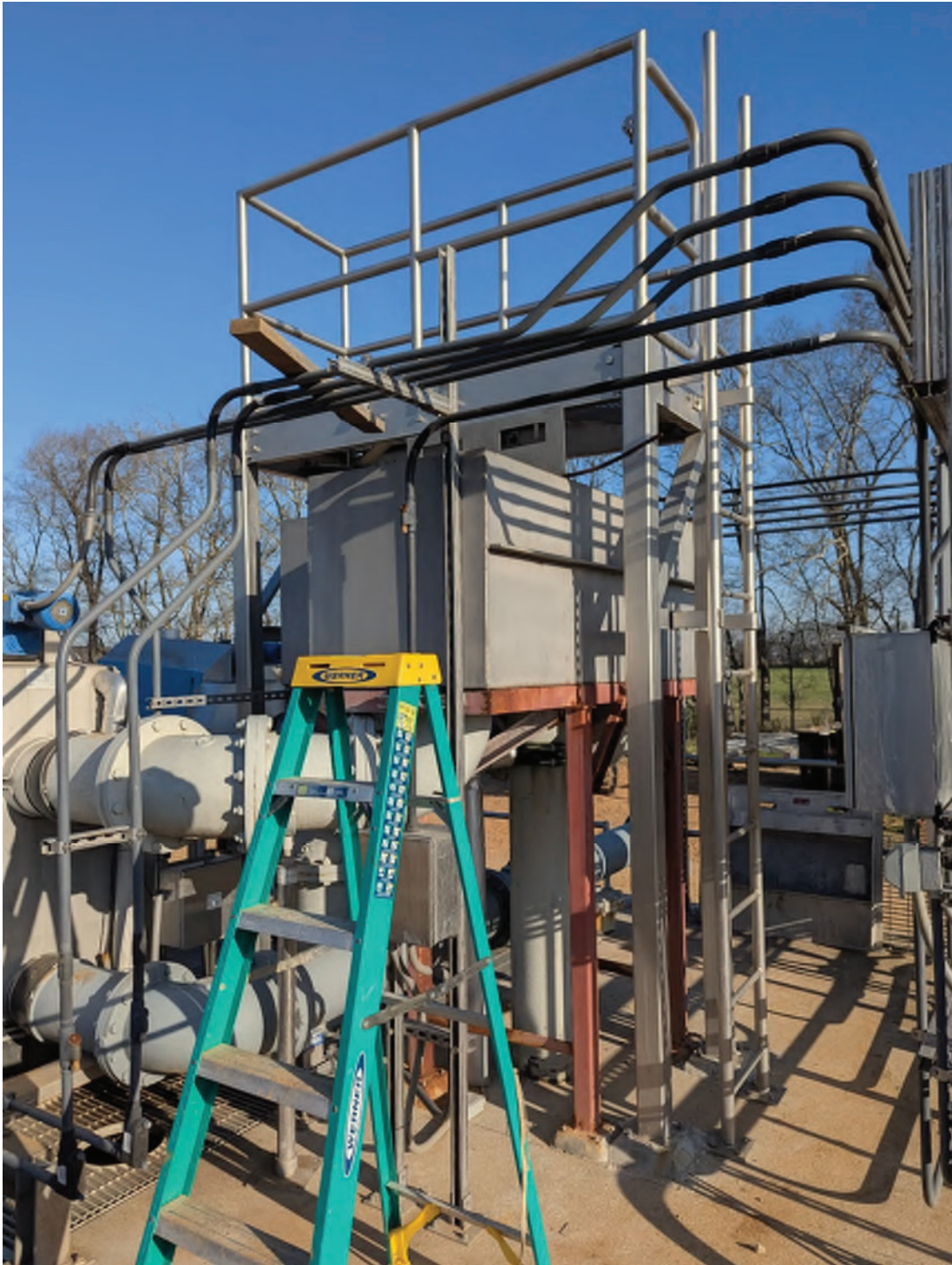
2. Headworks access structure
