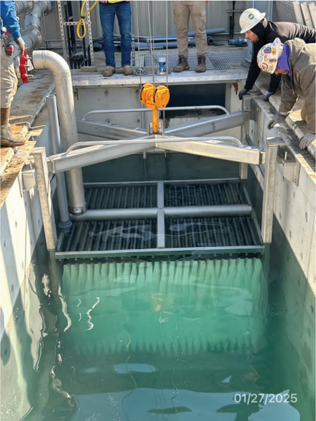
5. New membrane cassettes being installed.
