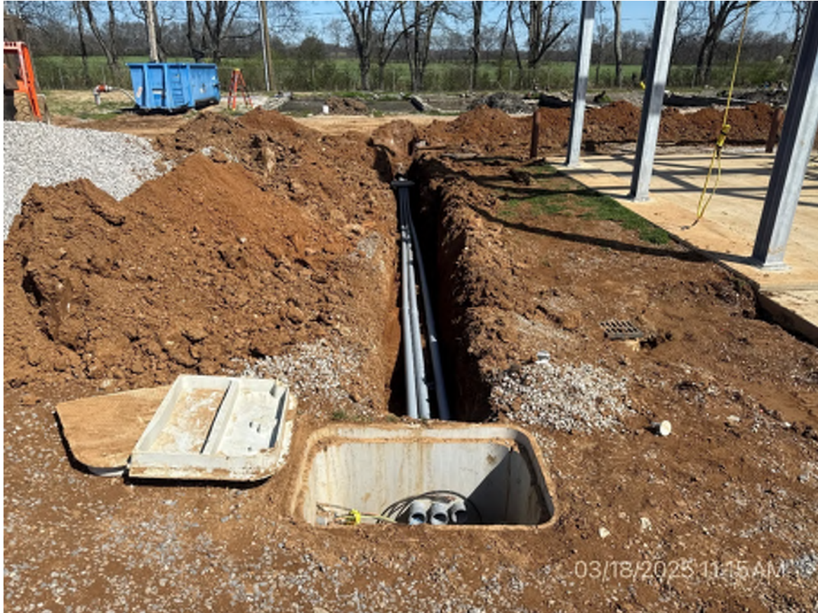
1. Conduit/Pullboxes Installed
