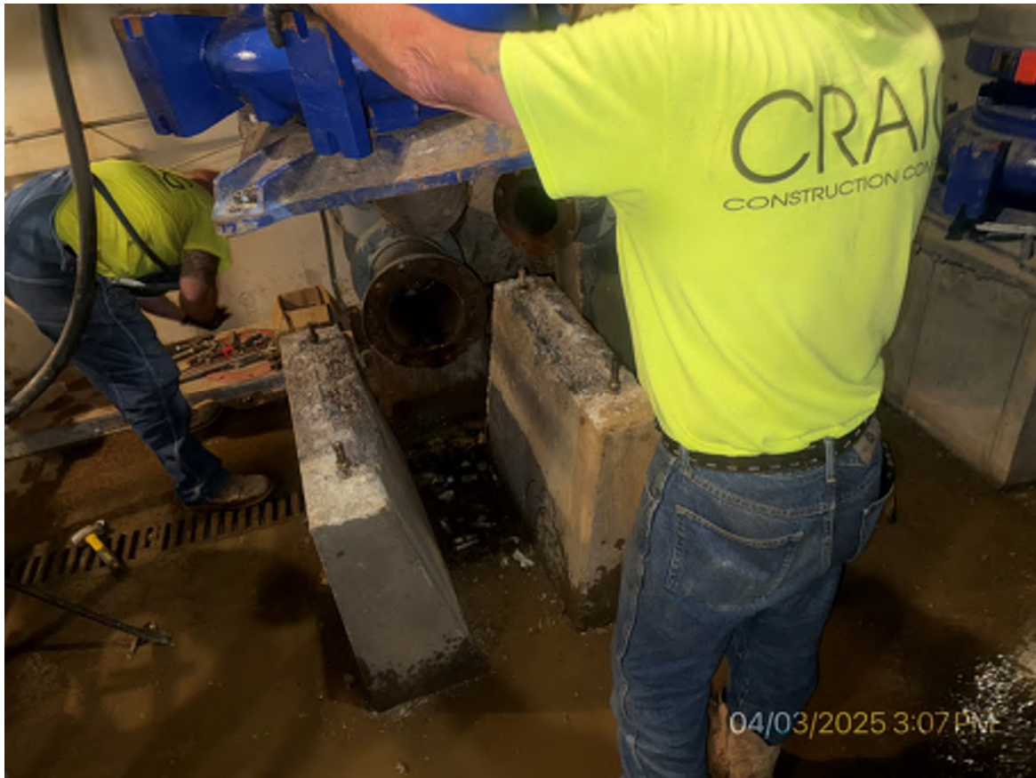
4. Installing final influent pump.
