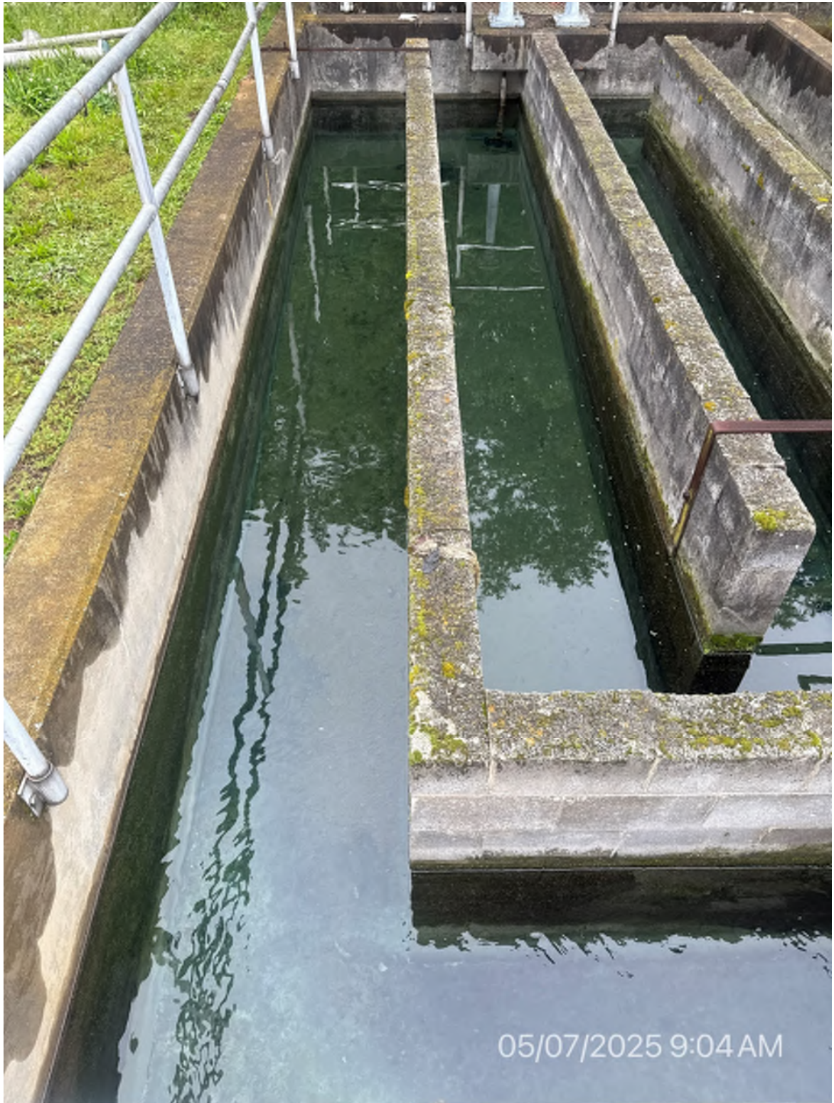
7. Effluent from MBR system in chlorine contact basin
