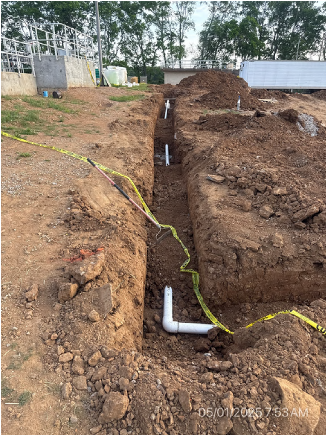
5. Installing chemical piping.
