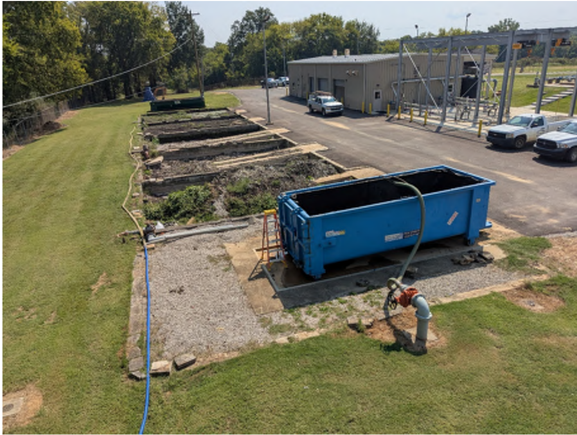
6. Sludge dewatering box and drying beds
