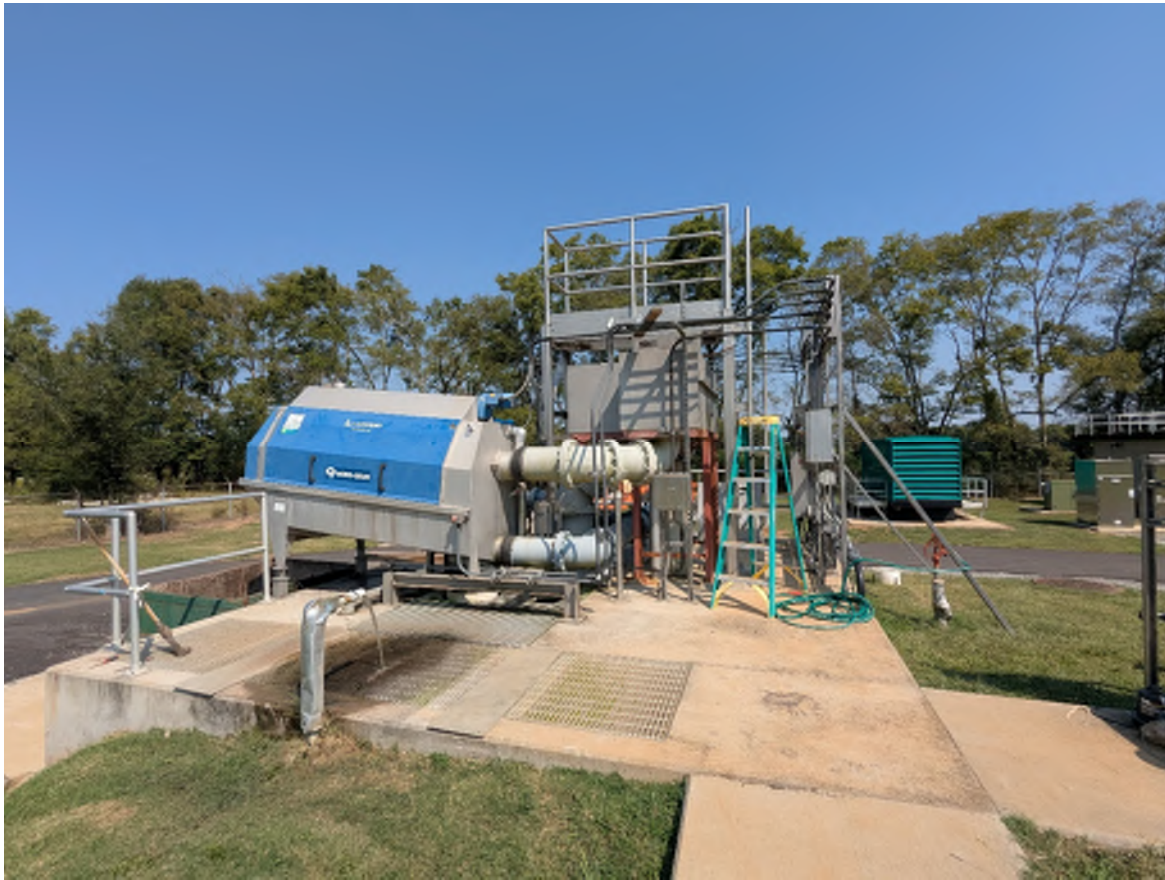
3. Headworks with fine drum screens
