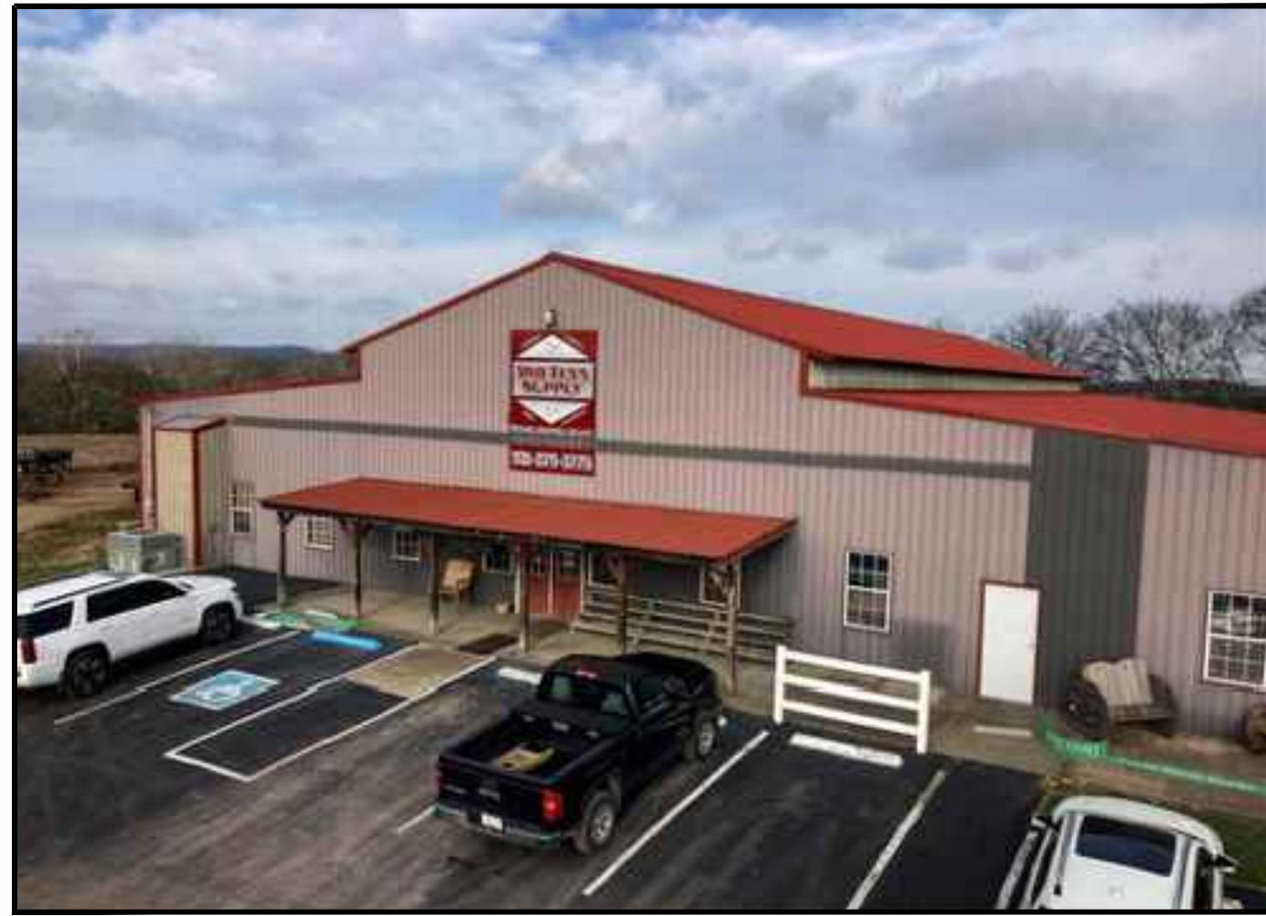
EXISTING PRINCIPAL STRUCTURE (BUILDING MATERIALS EXHIBIT)
