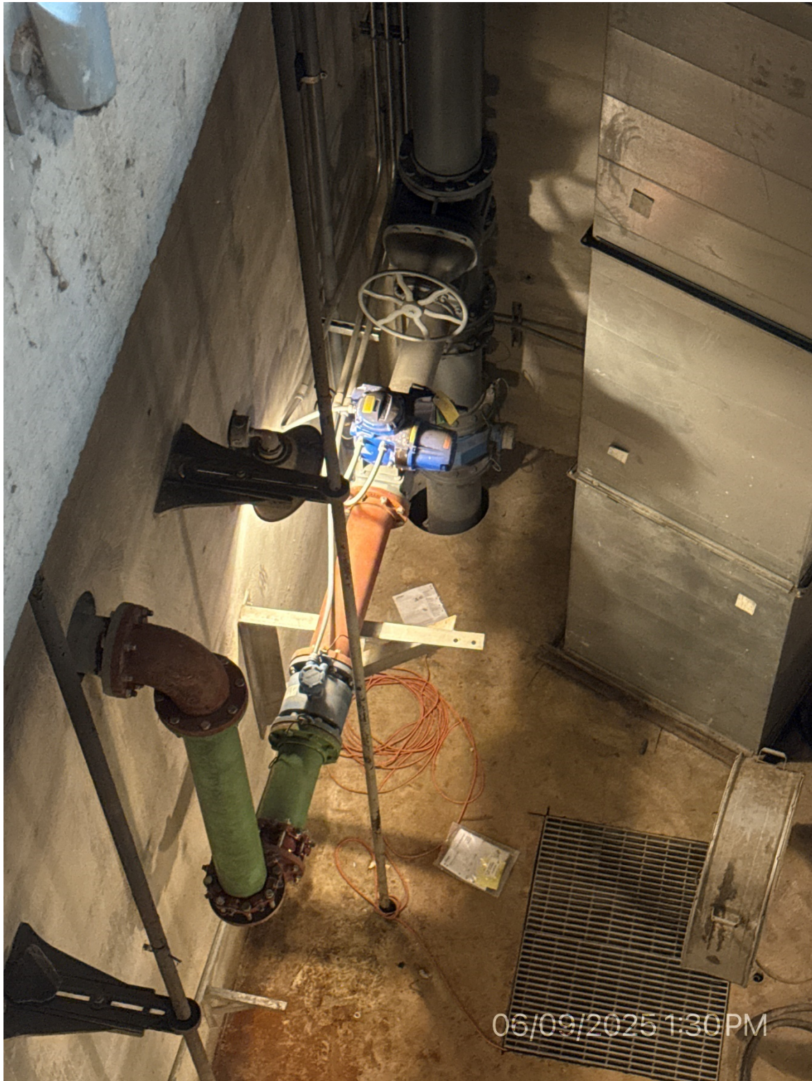
3. Installed Lagoon Return Piping
