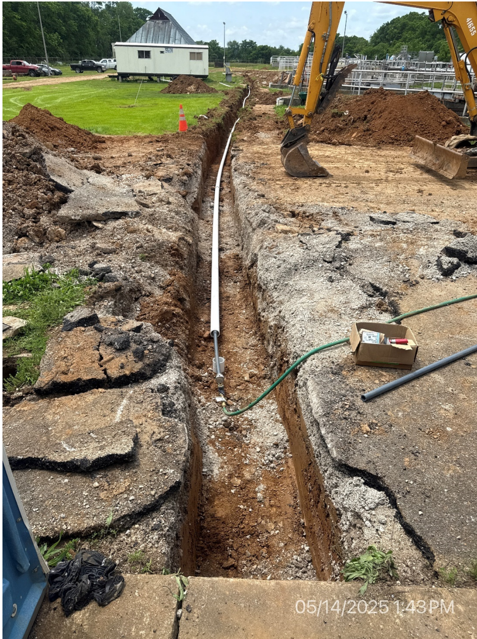
5. Installed Future Chemical Feed Piping
