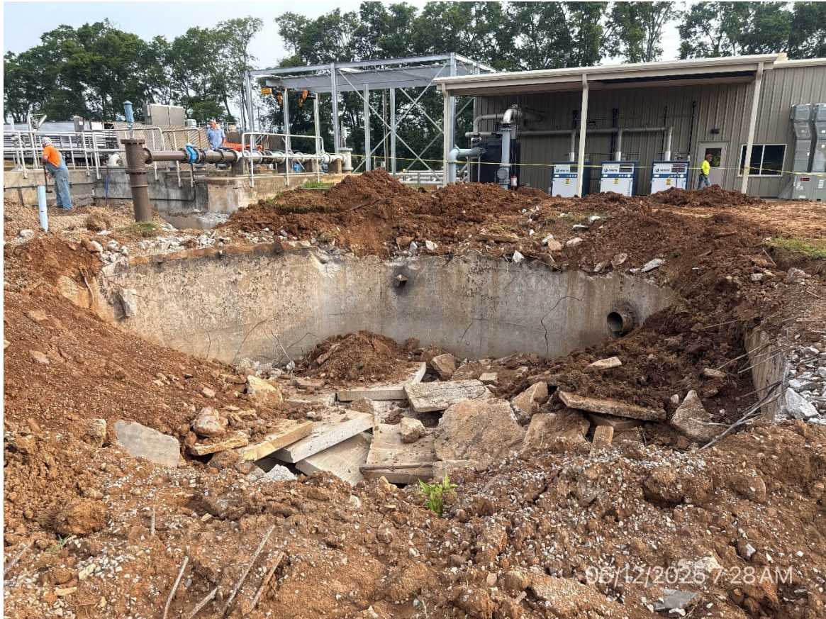
6. Demolition of Secondary Clarifier
