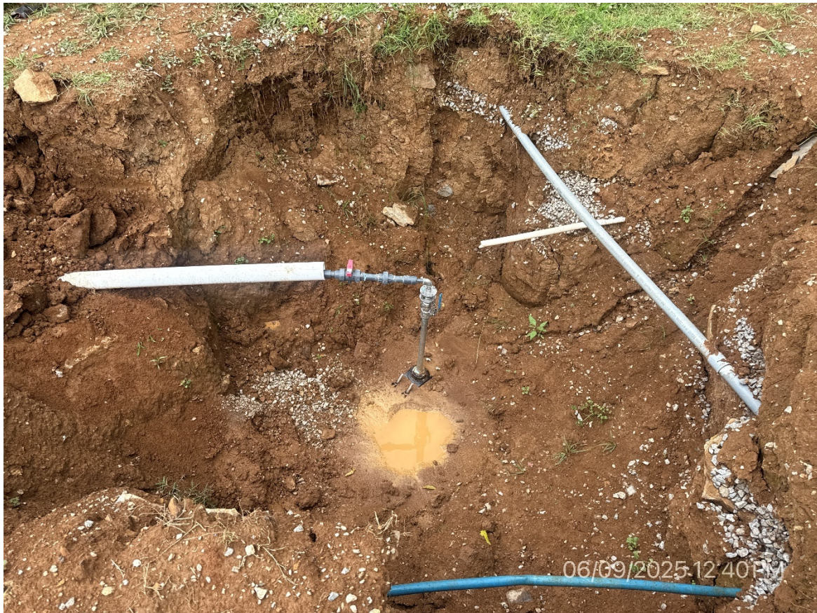
2. Installing Future Chemical Injection
