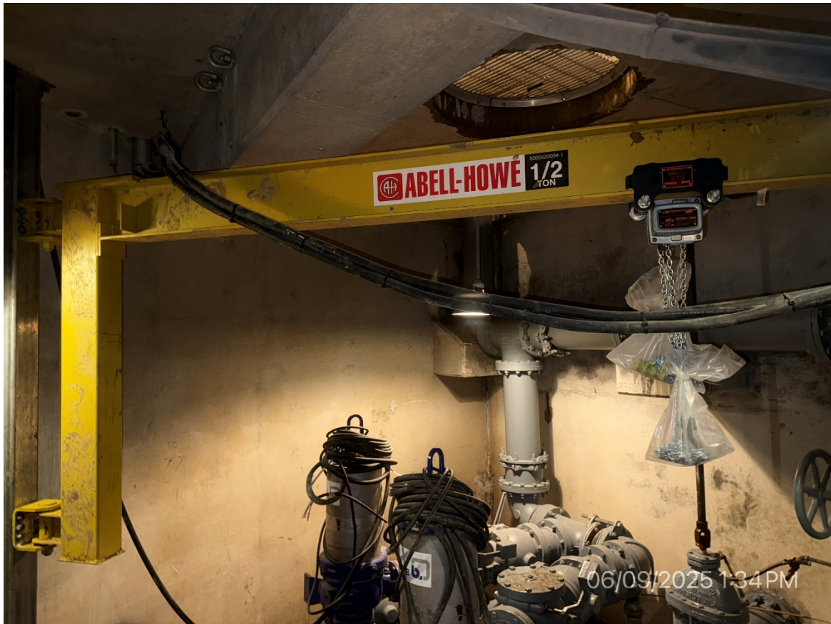
4. Installed Jib Crane at Influent Pump Station
