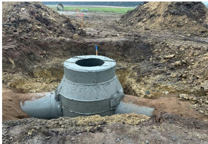
August 25, 2025 Sanitary Sewer Manhole Installation
