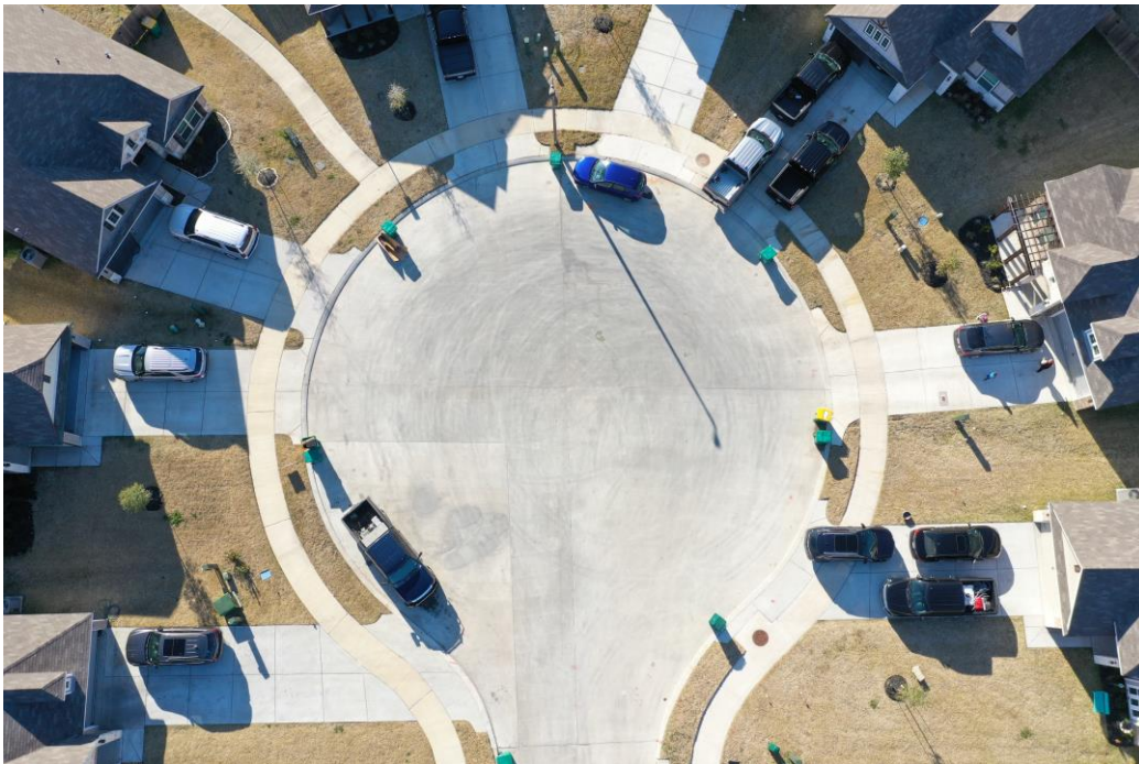
48 hours post- flooding (Post Repair)
