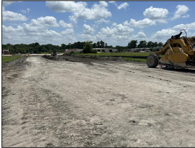
July 15, 2024 Subgrade Preparation
