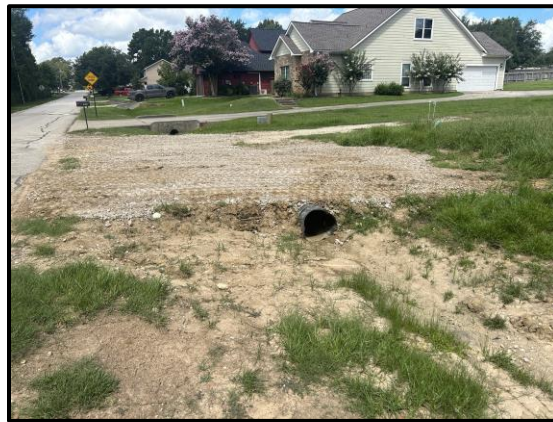
June 24, 2024 Trench Backfill & Driveway Restoration
