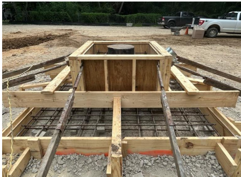
Well Pump Foundation Formwork
