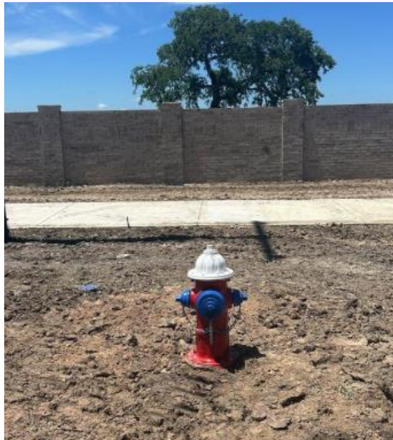
July 24, 2025 Installed Public Fire Hydrant
