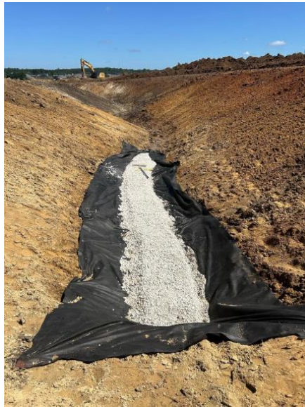
July 24, 2025 French Drain Installation
