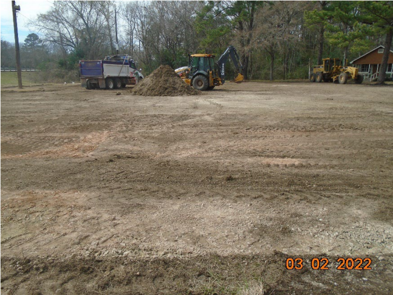
Scraping the old material from the site.
