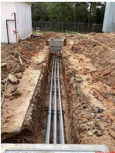
Figure 1: Electrical conduit installation October 18, 2022
