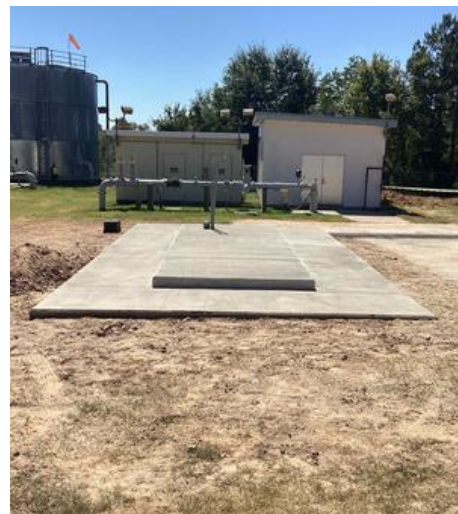
Figure 2: Newly constructed Generator Pad October 5, 2022
