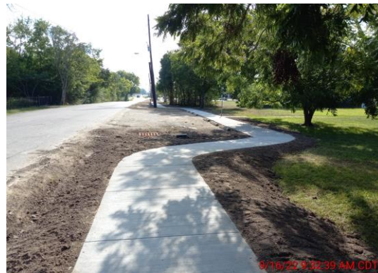
Figure 1: Newly constructed sidewalk September 16, 2022
