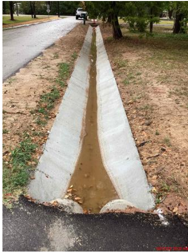
Figure 1: Newly constructed roadside ditch October 17, 2022
