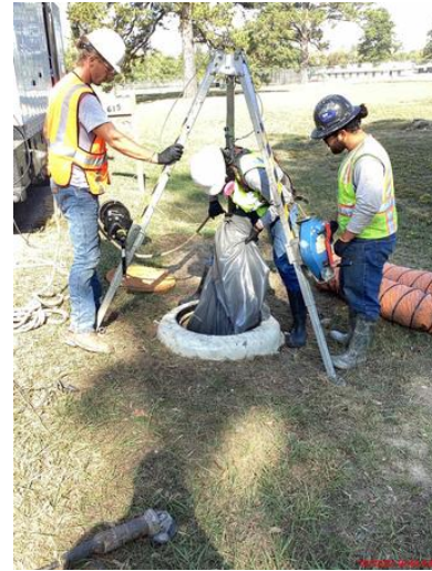
Figure 2: Manhole rehabilitation October 10, 2022
