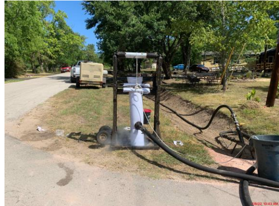
Figure 2: Sanitary Sewer CIPP Installation July 8, 2022
