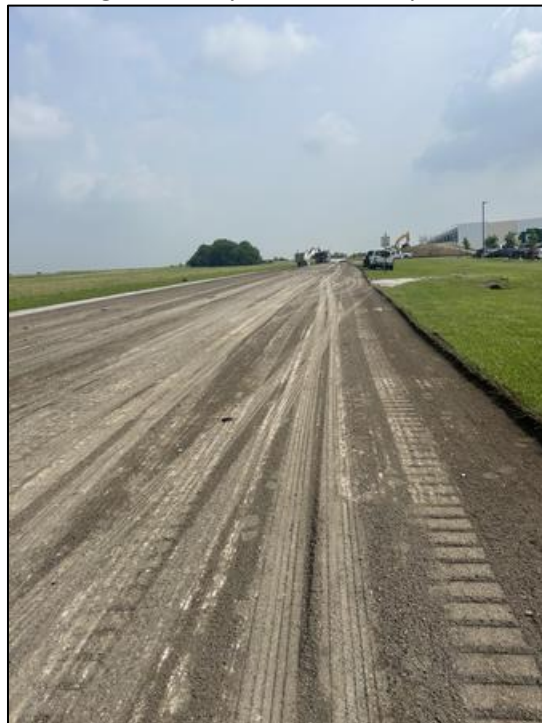
May 21, 2024 Existing Asphalt Removal
