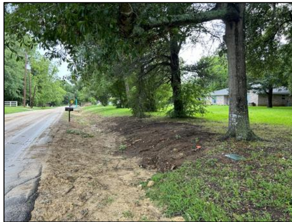
May 28, 2024 Trench Backfill
