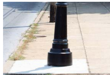
Acceptable Footer Detail
