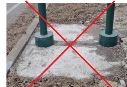
NOT Acceptable Footer Detail
