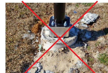
NOT Acceptable Footer Detail
