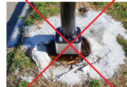
NOT Acceptable Footer Detail
