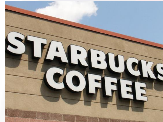
Example of a channel sign
