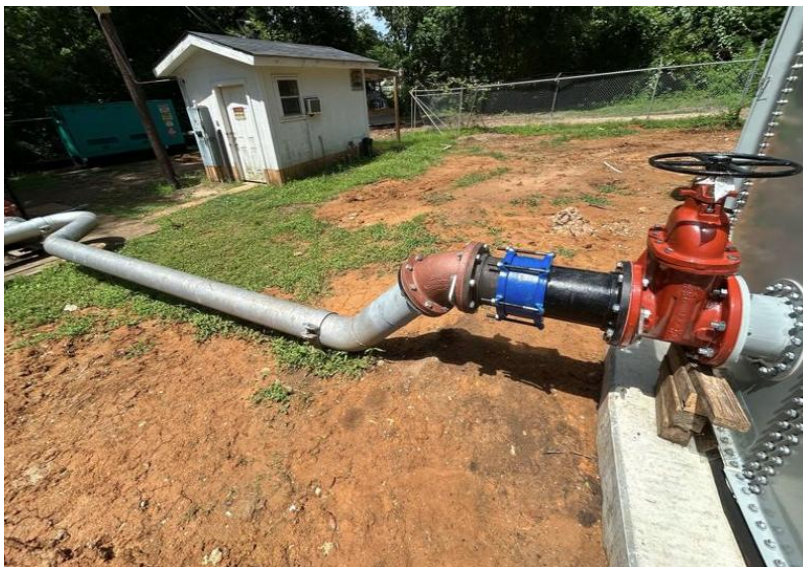
June 9, 2025 Feed Line into GST
