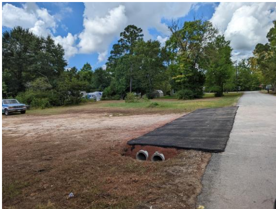
Figure 1: Culvert Replacement July 15, 2022
