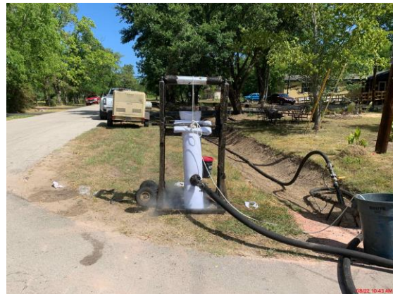
Figure 2: Sanitary Sewer CIPP Installation July 8, 2022
