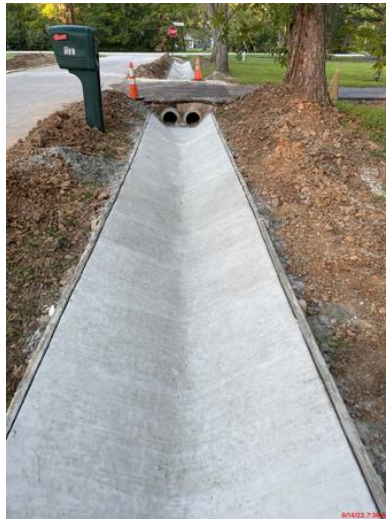
Figure 1: Newly constructed concrete lined ditch September 14, 2022
