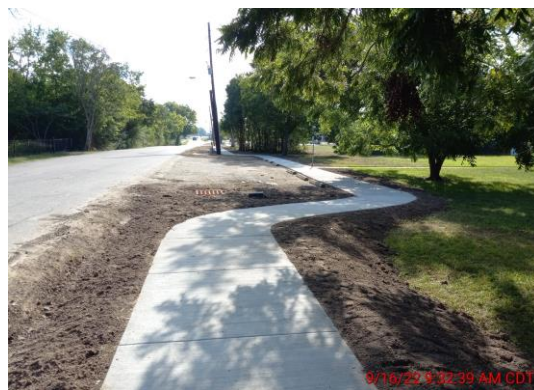
Figure 1: Newly constructed sidewalk September 16, 2022
