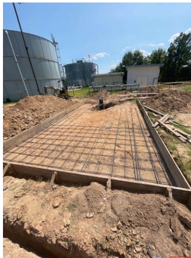
Figure 1: Generator pad formwork September 13, 2022
