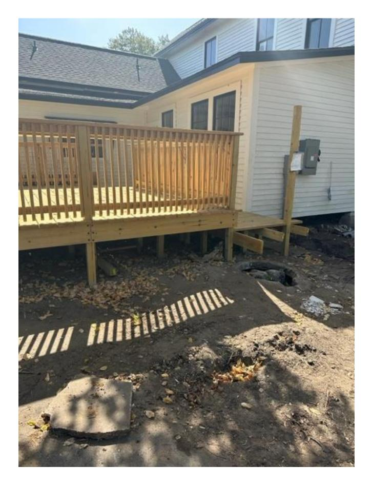
The entire deck was constructed with ground contact, rated pressure, treated wood.
