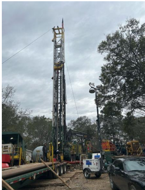
January 14, 2025 Drilling the New Well
