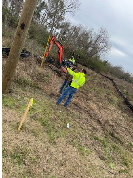
January 15, 2025 SWPPP Installation
