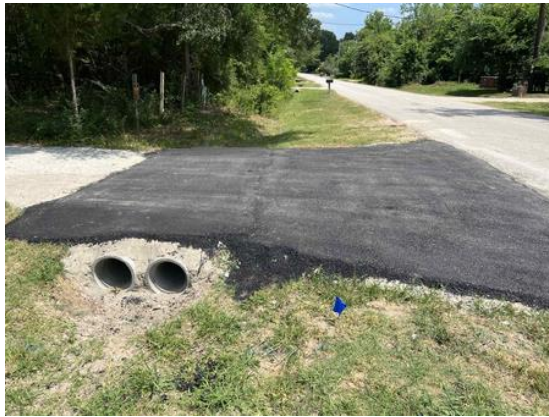
Figure 2: Culvert Replacement June 9, 2022
