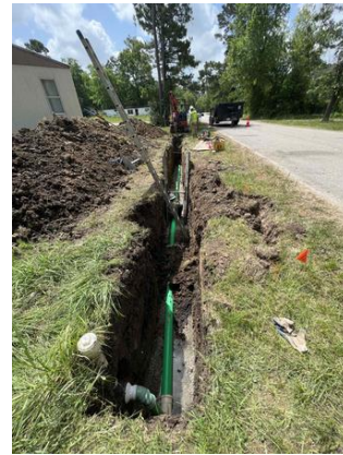
Figure 2: Sanitary Sewer Repair June 17, 2022
