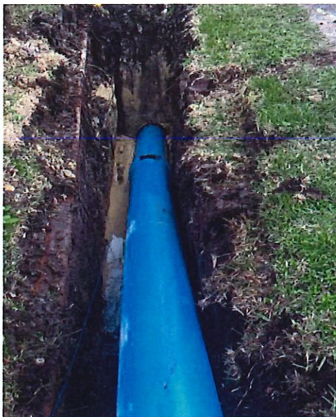
Trenchless construction on Pond St.
