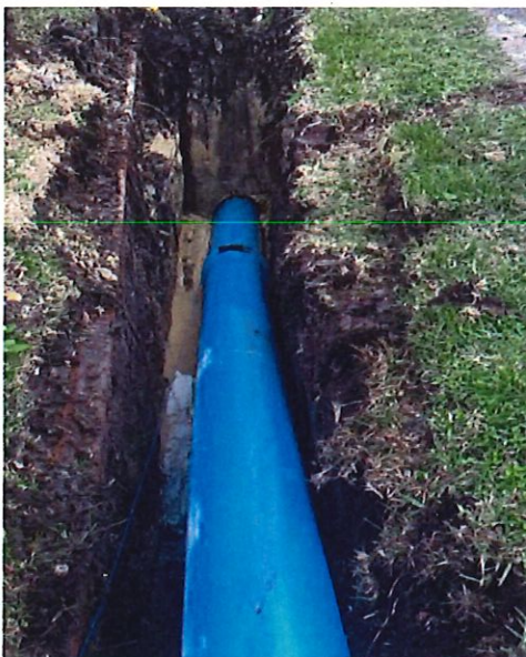
Trenchless construction on Pond St.
