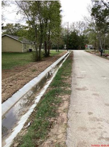
Figure 1: Newly Constructed Roadside Ditch along McGinnis November 15, 2022
