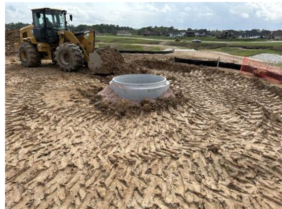
Installation of the Lift Station wet well October 25th
