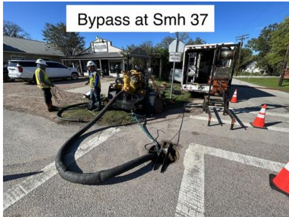
By-pass pumping at Sanitary Sewer Manhole No. 37 November 14 th
