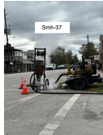
CIPP Lining at Sanitary Sewer Manhole No. 37 November 14 th
