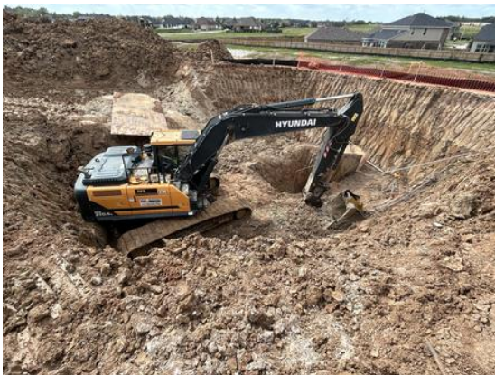
Excavation of the Lift Station wet well October 24th
