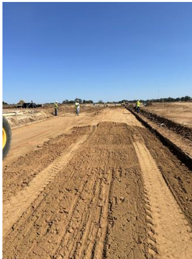
October 10, 2024 Roadway Grading
