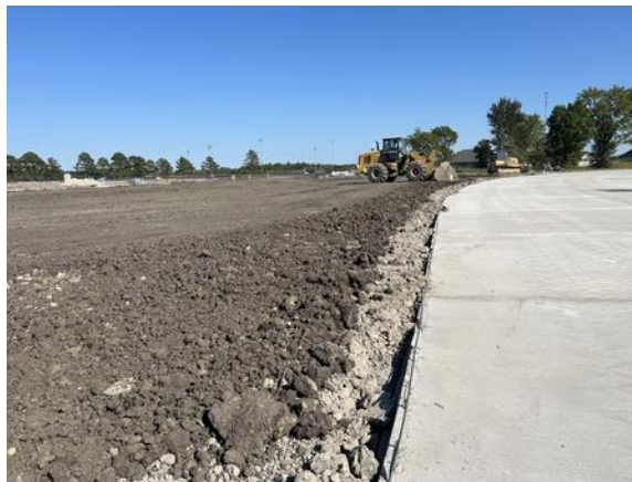
October 10, 2024 Residential Lot Grading
