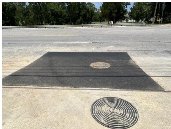
August 23, 2024 New Asphalt along SH 105
