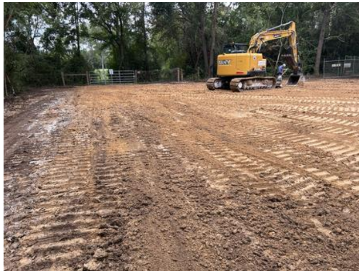
September 13, 2024 Water Plant Site Clearing
