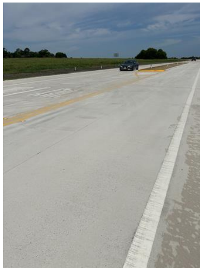
September 14, 2024 New Buffalo Springs Roadway
