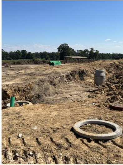
September 12, 2024 Cleared Site and Sanitary Sewer Installation
