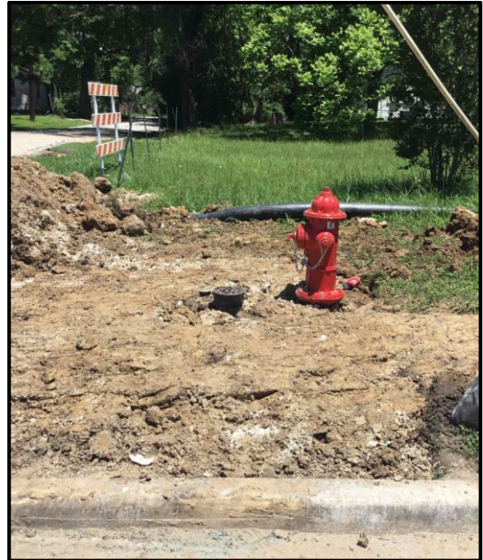
Flush Valve Install at SH-105 & Louisa St.
