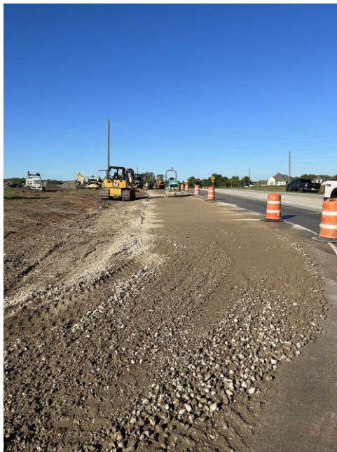
Subgrade Preparation (Westbound) October 18, 2023
