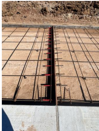
Formwork for proposed roadway February 9 th
