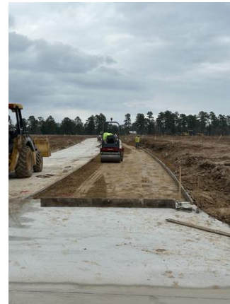
Roadway Compaction February 9 th
