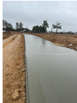
Formwork for proposed roadway January 18 th
