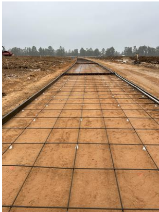
Formwork for proposed roadway January 18 th
