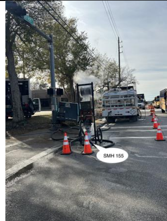
CIPP Lining along SH-105 on December 12 th
