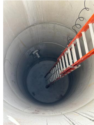
Inside Lift Station wet well January 17 th
