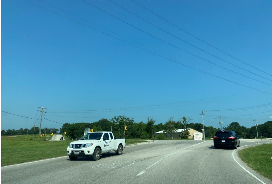
Figure 6 – FM 1097 at Buffalo Springs Drive Northbound Approach
