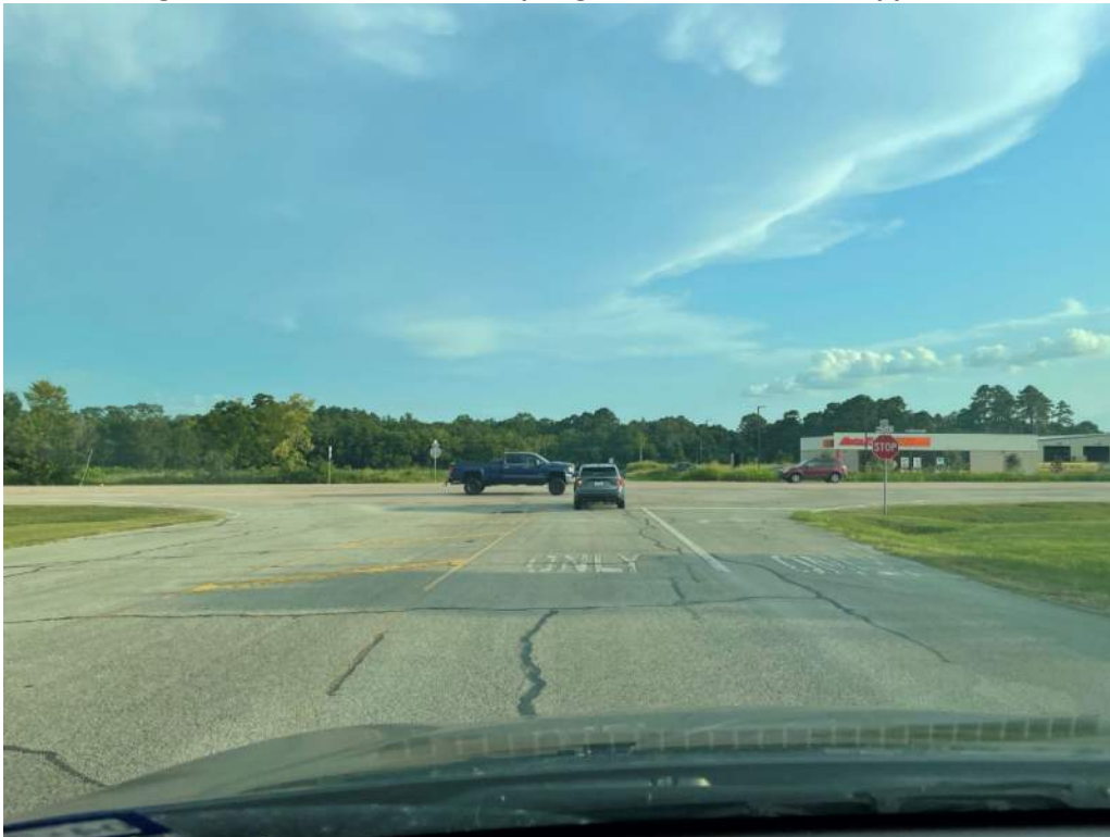
Figure 7 – SH 105 at Buffalo Springs Drive Southbound Approach
