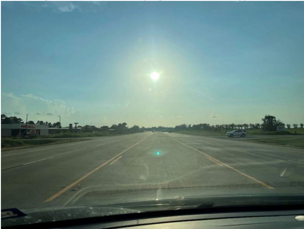
Figure 5 – SH 105 at Buffalo Springs Drive Westbound Approach
