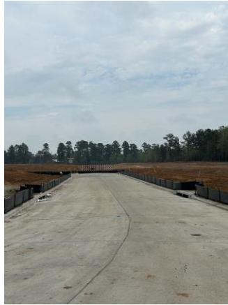
Roadway Paving March 15 th
