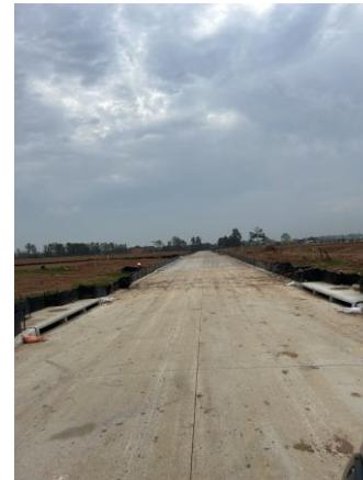
Roadway Paving March 15 th
