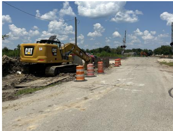
August 4, 2024 BNSF Railroad Bore
