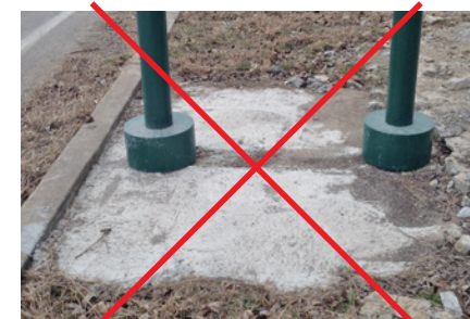
NOT Acceptable Footer Detail
