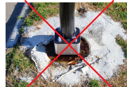
NOT Acceptable Footer Detail
