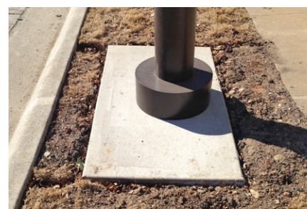
Acceptable Footer Detail
