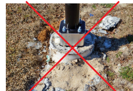
NOT Acceptable Footer Detail
