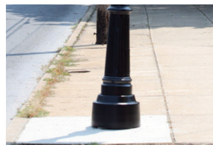
Acceptable Footer Detail
