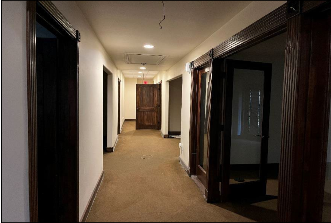
Interior view of the office area
