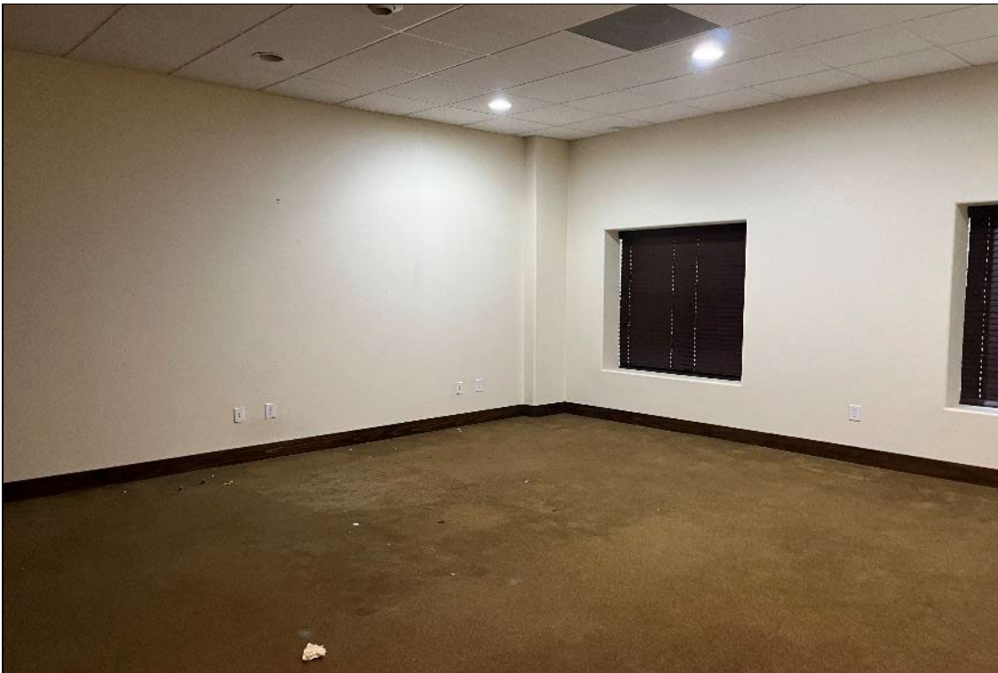
Interior view of the office area
