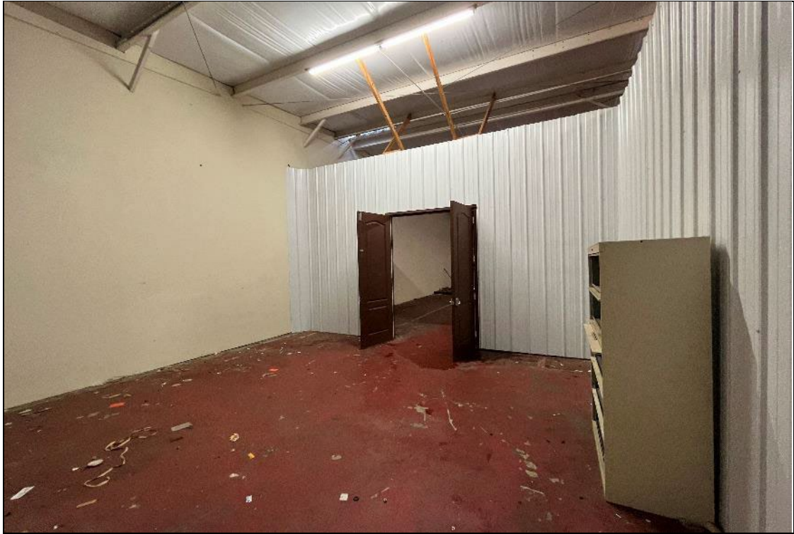
Interior view of the warehouse area
