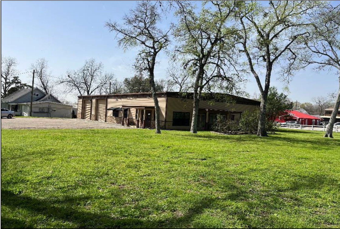
Exterior view of the subject building
