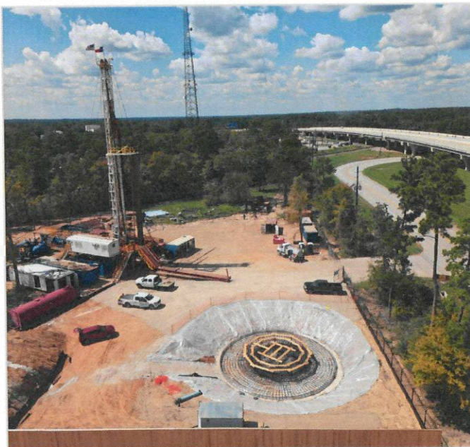
Drone imagery of the construction site of Water Plant No. 4 500,000-gallon Elevated Storage Tank (EST).
